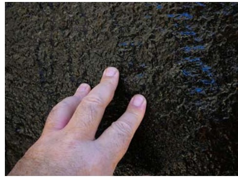
After 2 coats of Feronite Rusty Metal Primer
