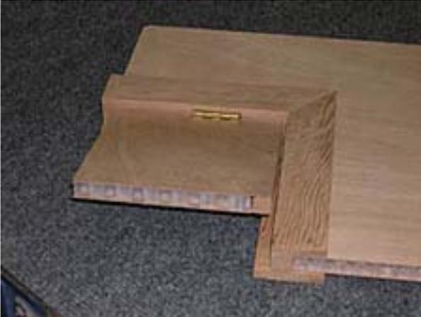
You can also make a frame for the door as in figure 15, and hang as normal.
